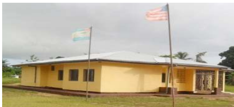
Newly constructed bank
